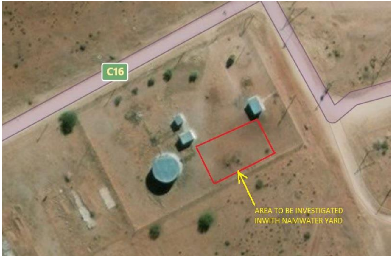
Figure 1 Aerial view of the Aroab NamWater Premises and Proposed Reservoir Location
