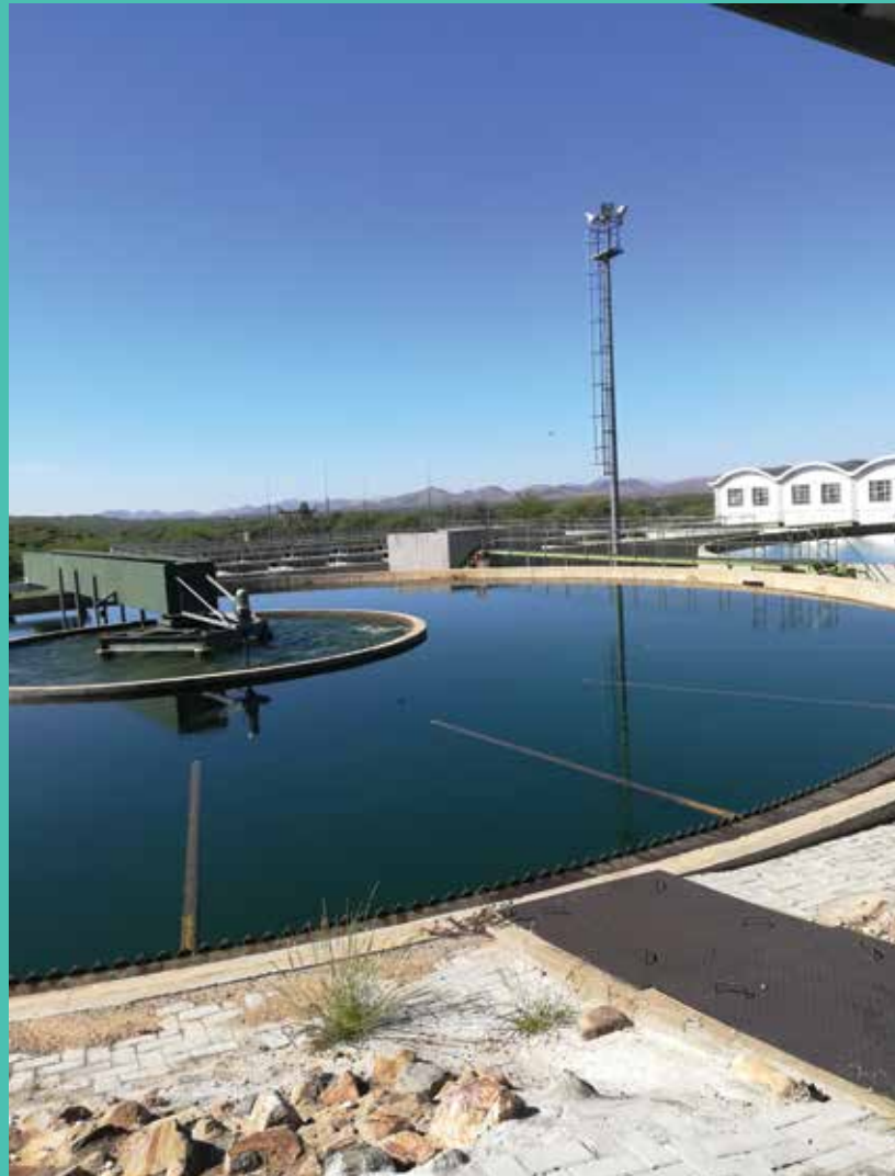
Clarifiers at Von Bach Purification Plant.
