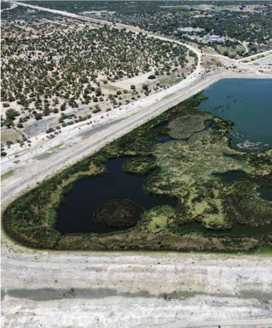
Ogonog Million Dam.
