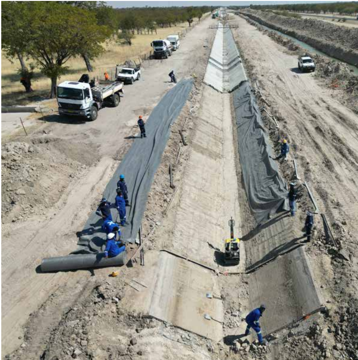
Calueque – Oshakati canal rehabilitation in progress.
